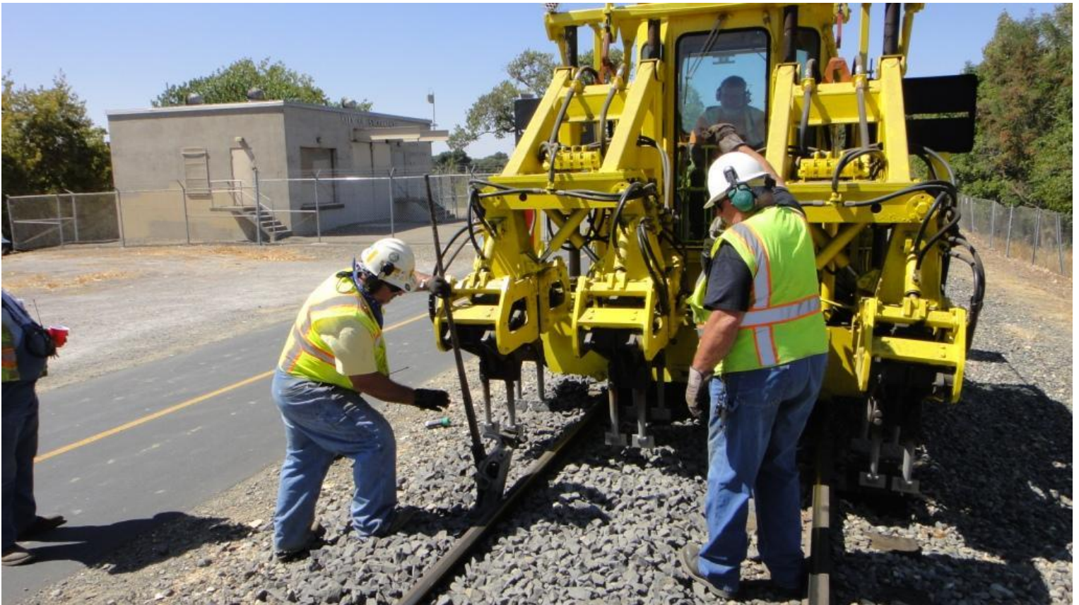
Harry gives Frank in the tamper a "stop" signal as Mike F. removes a jack
