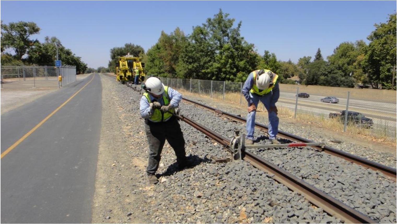
Heather jacks a track-jack as Alan checks the level
