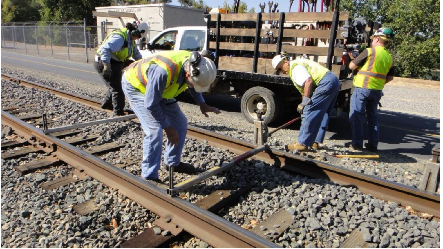
Clem jacks the track-jack as Alan monitors the level
