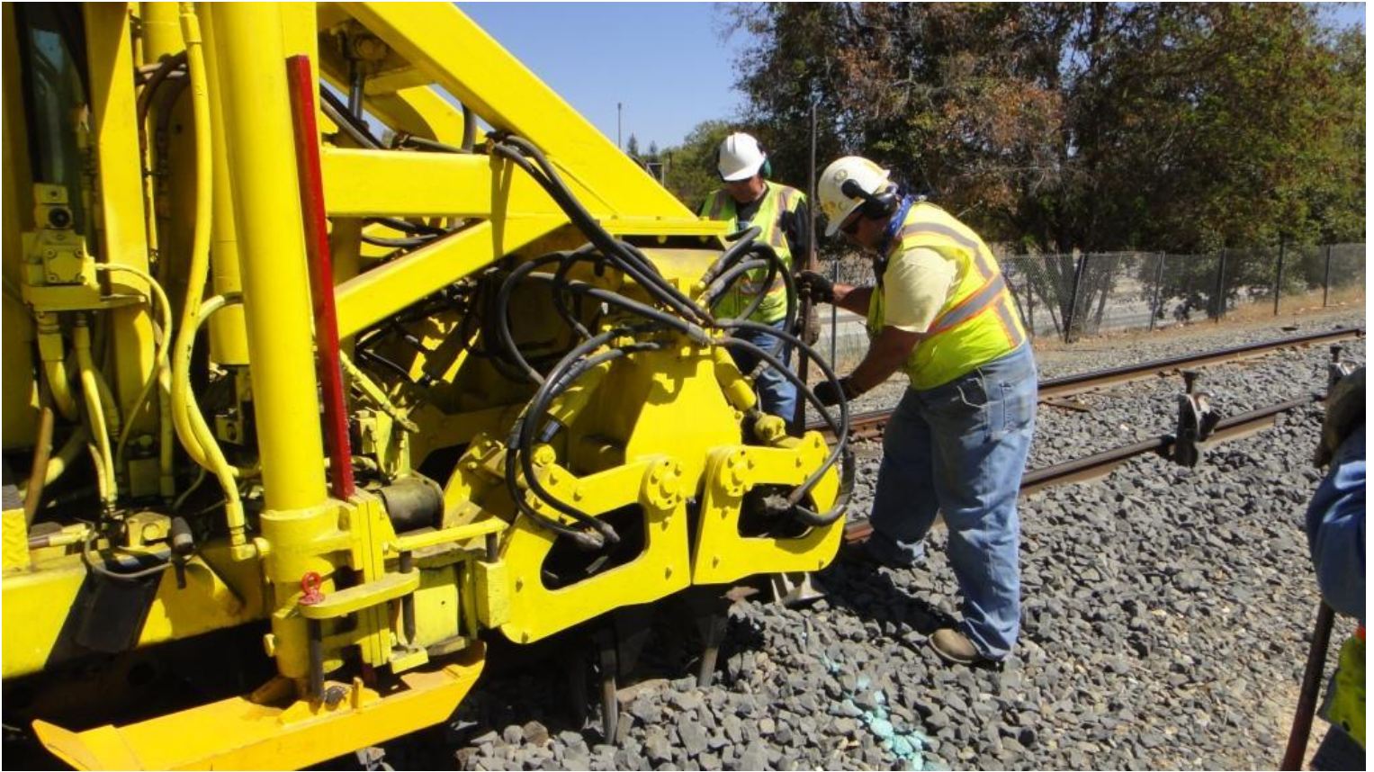
Mike F. pulls a track-jack as the tamper approaches
