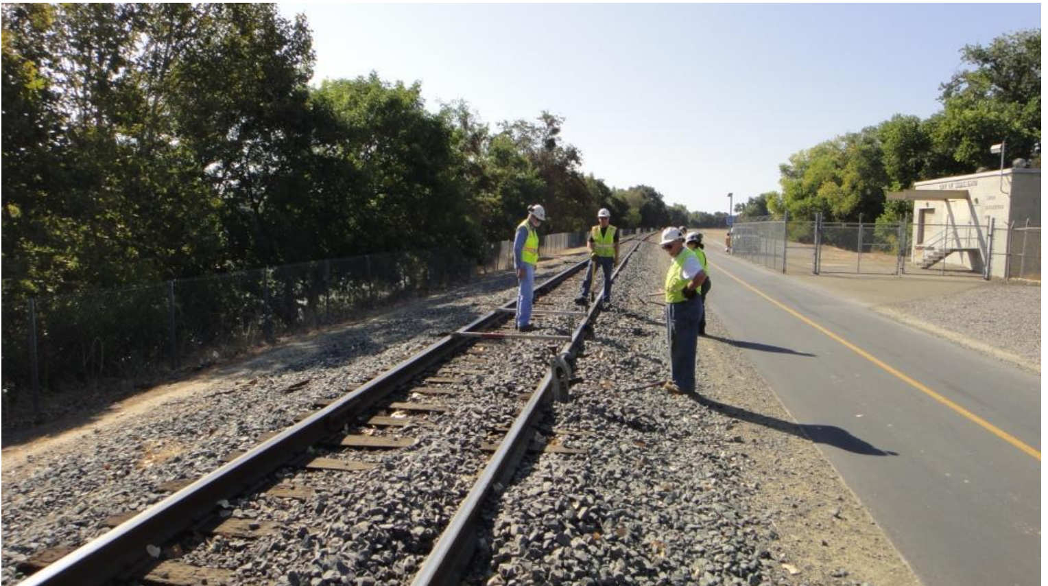
At MP 3.6, as the track-jacks are set, track-levels are placed on the track to guide the raise of the west rail
