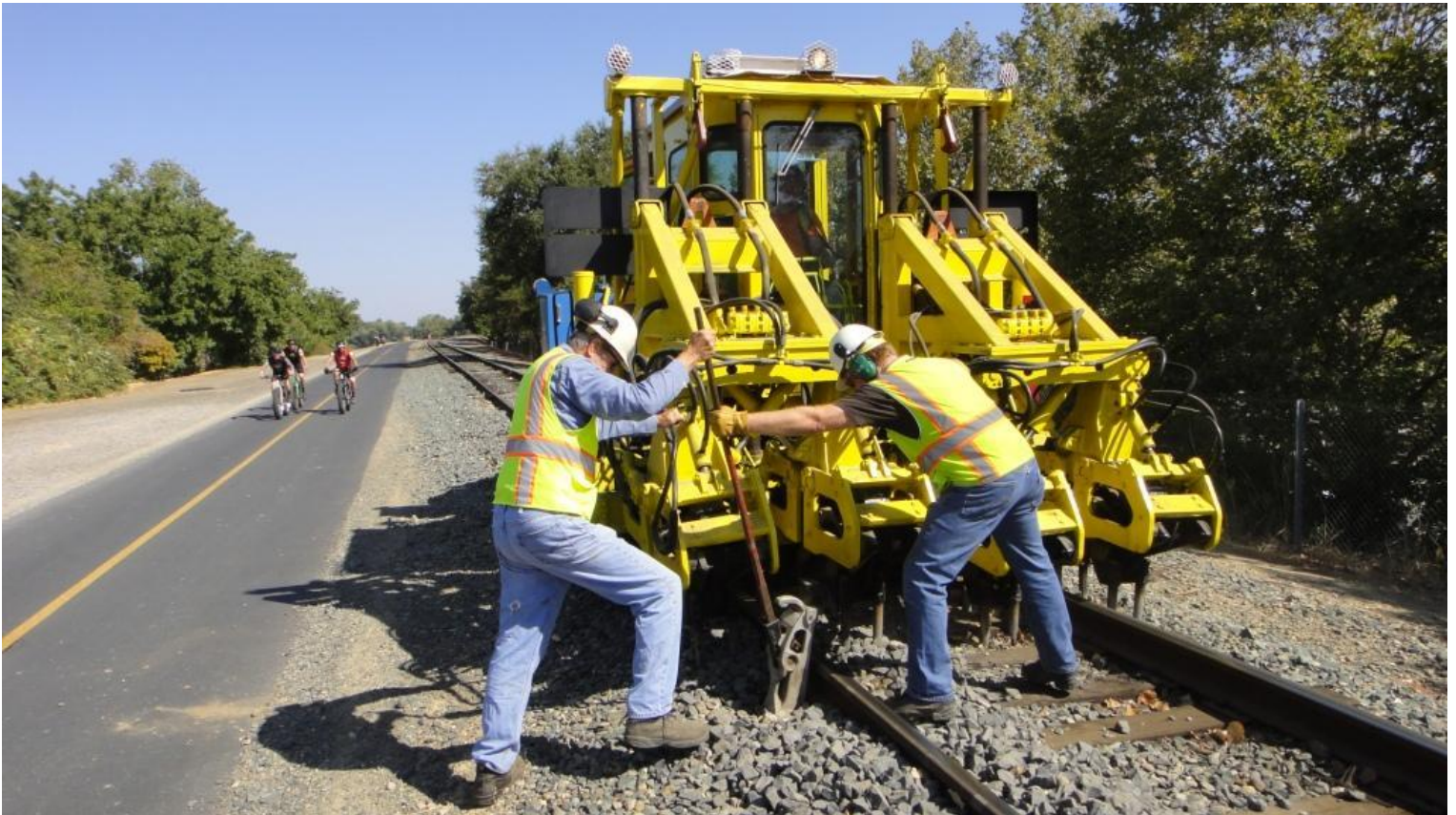
Alan and Ed struggle to remove a track-jack as the tamper approaches
